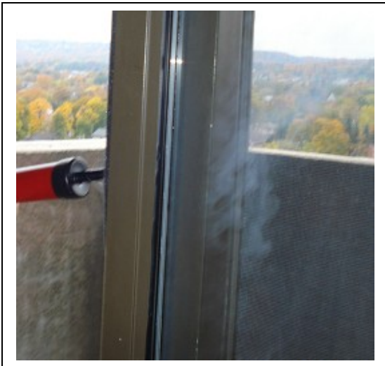
Smoke blown inside a door appears outside.
