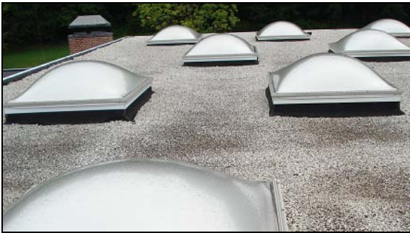
Skylight perimeters should be sealed.
