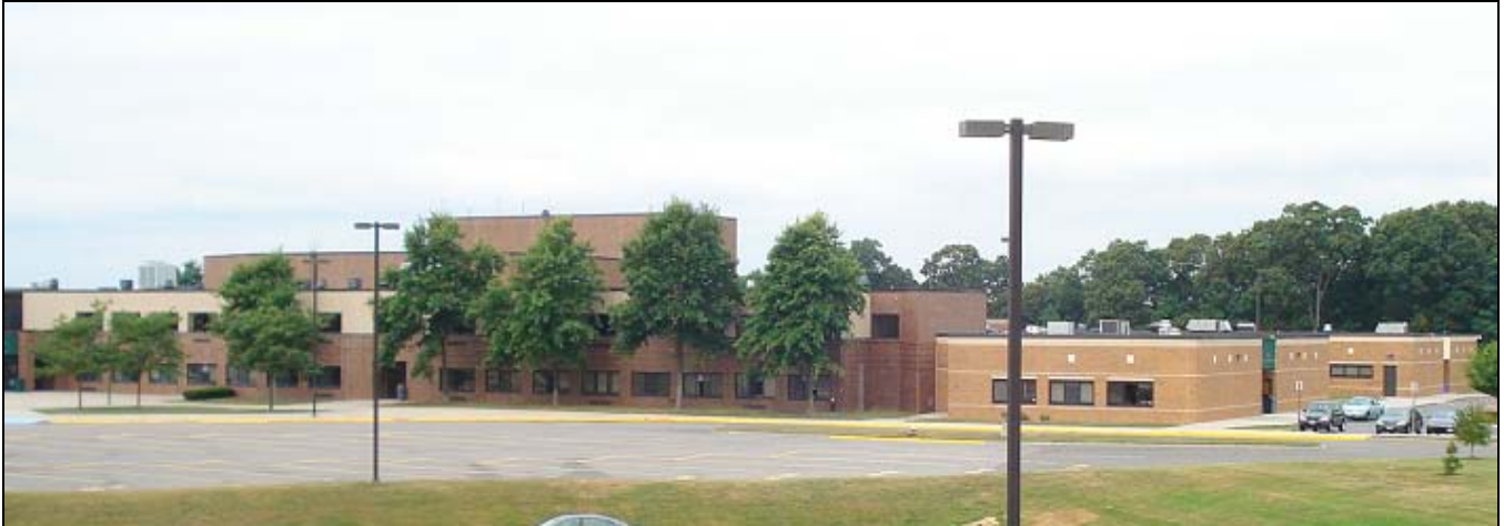
Originally built in 1985, an addition in 2006 expanded the building's size to 550,000 square feet.
